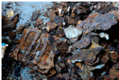
Iron Chips from poor lay-up will clog strainers and tower nozzles, reducing flow and increasing head pressure
